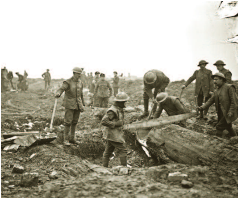
Pioneers removing tree stumps in preparation for track laying (© IWM Q 8401)
